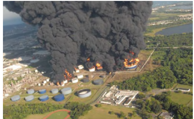
Figure 11: View of Terminal Day after Incident
