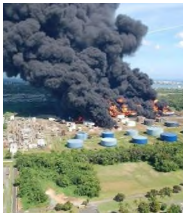
Figure 15: Results of Vapor Cloud Explosion
