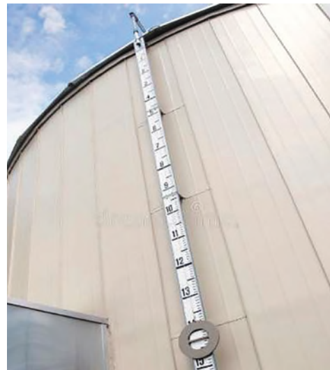
Figure 26: Example of a Tank Gauging System
