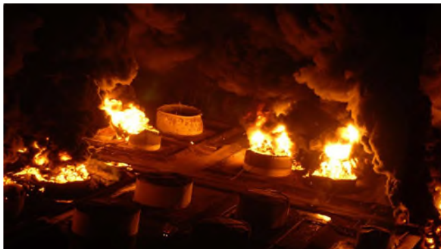
Figure 10: 2009 Capeco Tank Overfill Incident 7
