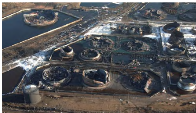
Figure 9: Buncefield after the Incident with the Culprit Tank T-912 Initiating Event at Center Foreground 6
